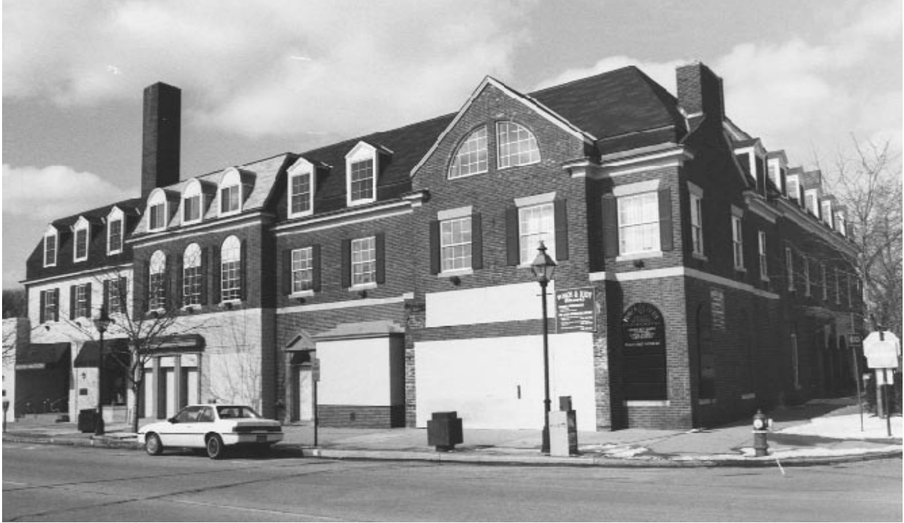
Punch and Judy Building under renovation, 1987.
